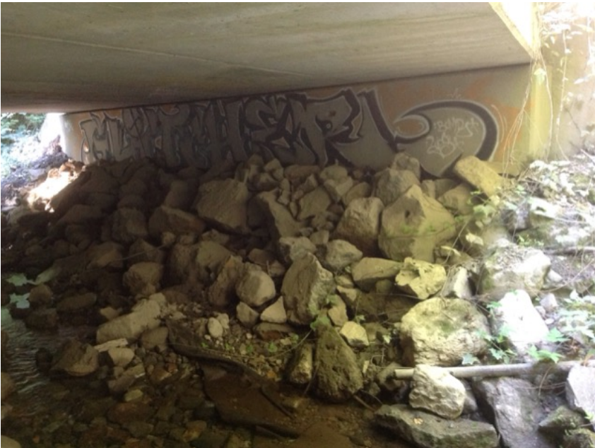
Right Bank Abutment when facing downstream
