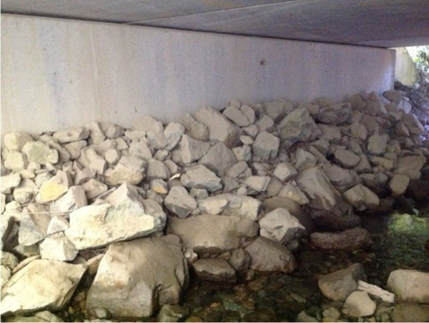
Left Bank Abutment when facing downstream
