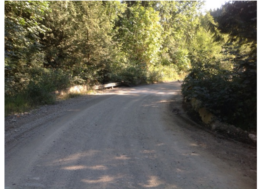
Approach from Right Bank when facing downstream
